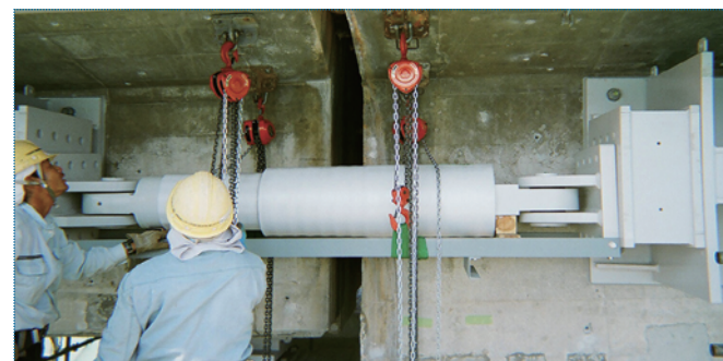
Site Installation (PC Bridge)
