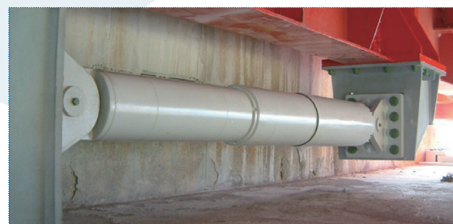
Site Installation (PC Bridge)
