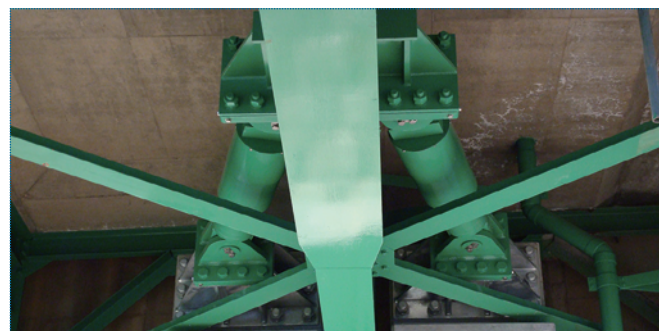
Site Installation (Steel Bridge)
