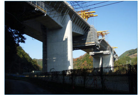
ASAHINA VIADUCT in the 2nd Tomei Expressway
