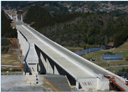
OIDAIRA VIADUCT in the 2nd Tomei Expressway
