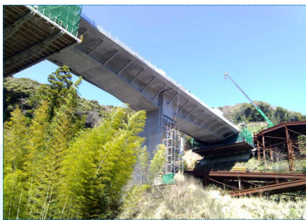
OGAWA 1st BRIDGE in the 2nd Tomei Expressway
