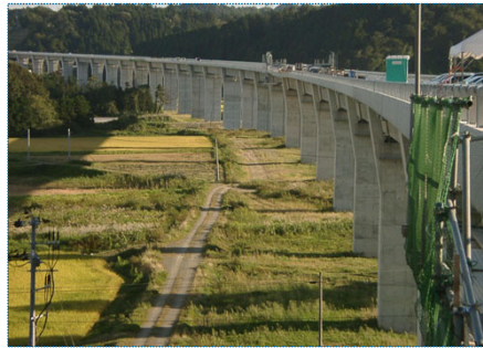
KIDOGAWA BRIDGE in the Jyoban Expressway
